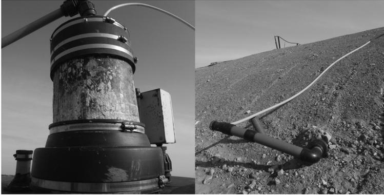
*Photo 5. Gas wells on the Hill of Tramaud landfill.*
